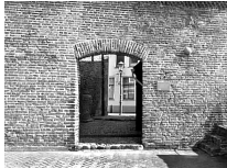
Figure 3 This a gate.
